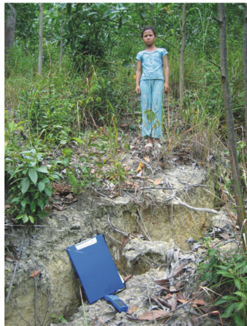
Fig. 13 Signs of potential landslides in Van Canh district (tension crack and scarp at the top)
