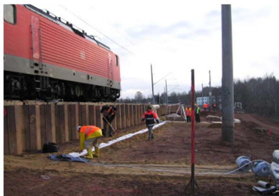
Fig. 17 Installation of sensor-equipped geotextiles in a railway embankment in Saxony/Germany [11].
