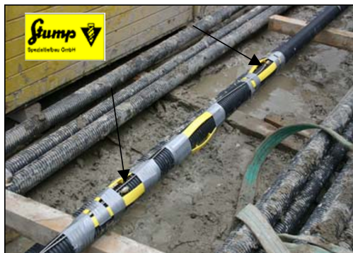
Fig. 21 Prefabricated anchors with fixed pH sensors (arrows).
