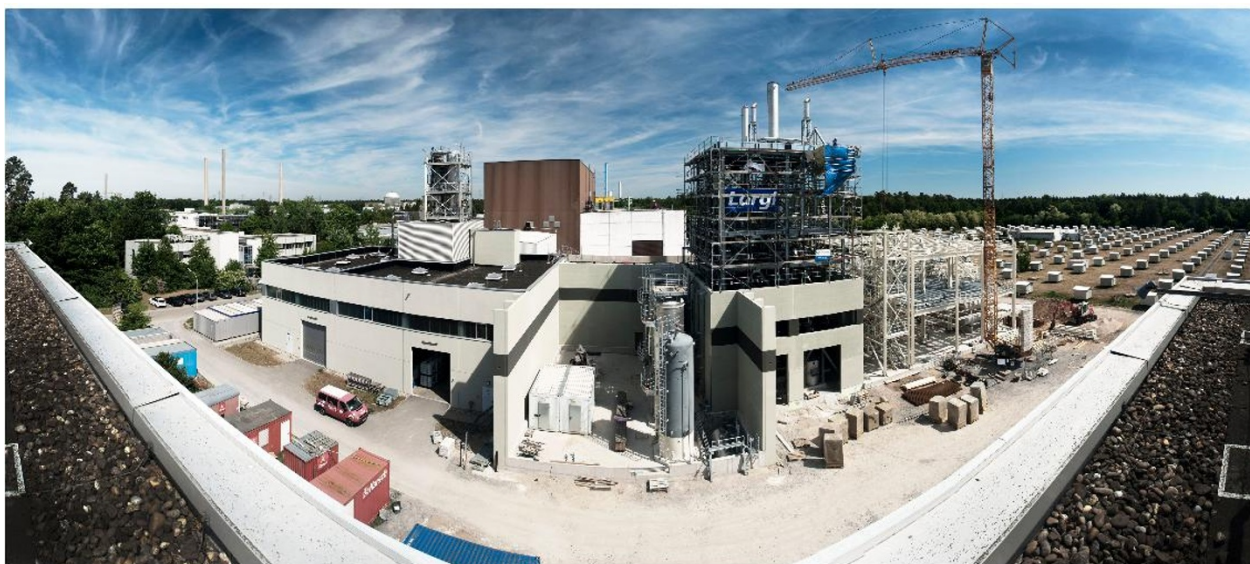
Figure 5 The bioliq ® pilot plant construction site.
