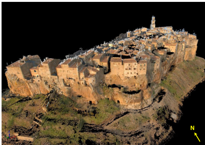
Fig. 4 Holistic true coloured point cloud of the Pitigliano cliff and the historic centre
