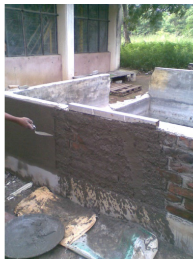
Fig. 6 Plastering of vertical surface of brick masonry wall
