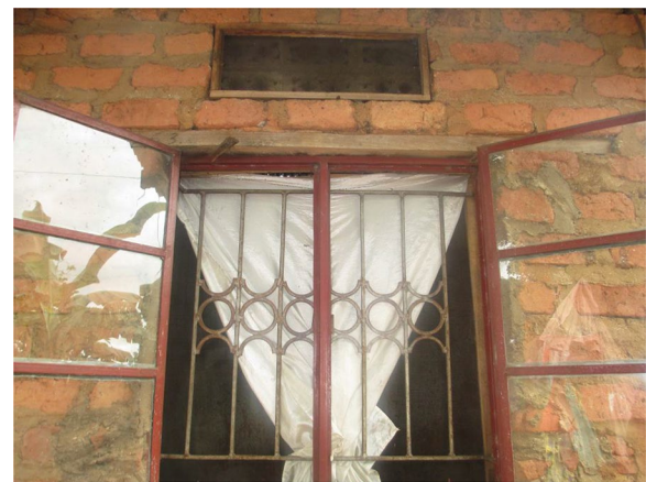
Fig. 3 A window and ventilator with screening on one of the demonstration houses
