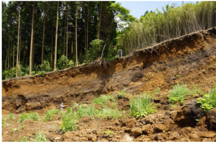
Fig. 15 Soil layers in the right flank of the landslide
