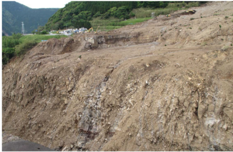
Fig. 10 Highly weathered bedrock at the foot of the Aso Bridge landslide
