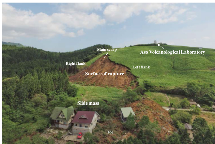
Fig. 14 Aerial view of the landslide near Aso Volcanological Laboratory
