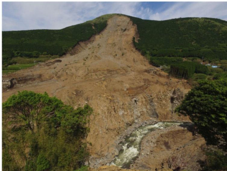
Fig. 5 The front view of Aso Bridge landslide
