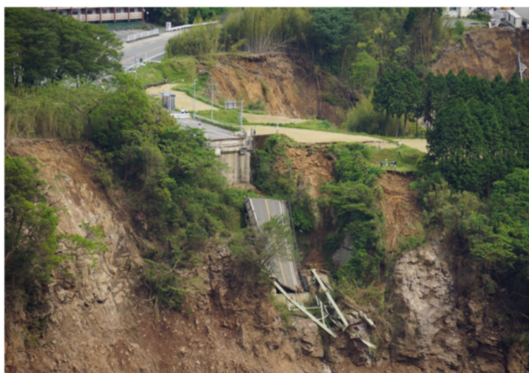
Fig. 7 The Aso Bridge tumbled into the Kurokawa River after the landslide event
