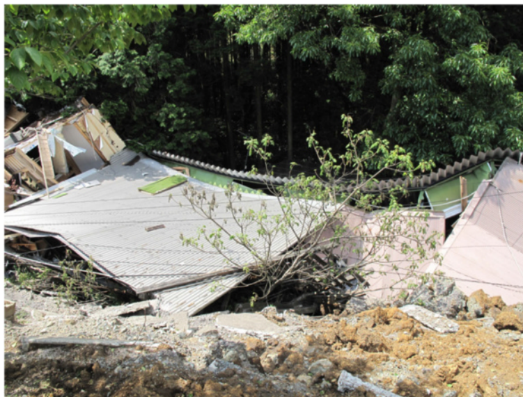
Fig. 16 Collapsed wood-frame houses at the toe of the landslide
