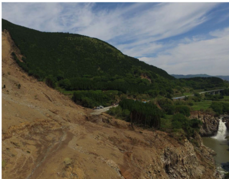
Fig. 8 The road buried by the displaced mass
