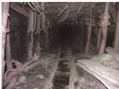
Fig. 7 The appearance of panel 1111(1) roadway retention
