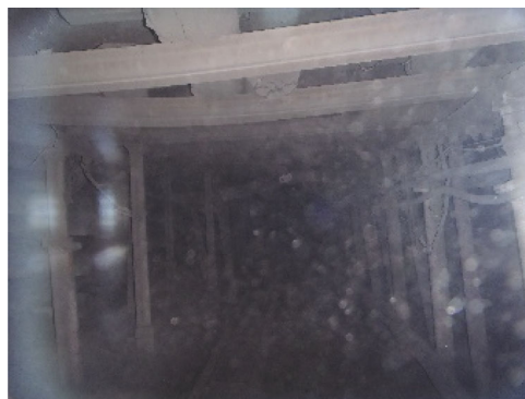
Fig. 10 The appearance of the working face 1112(1) roadway retention
