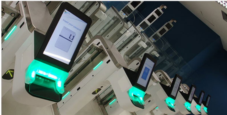
Figure 6.14: Electronic gates for the ABC control
