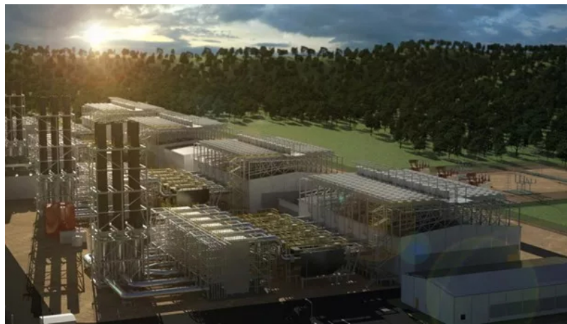
Figure 2. Battery of Boilers in a Combined Cycle Plant. The innovative way of heat optimization. (Wärtsilä, 2016)
