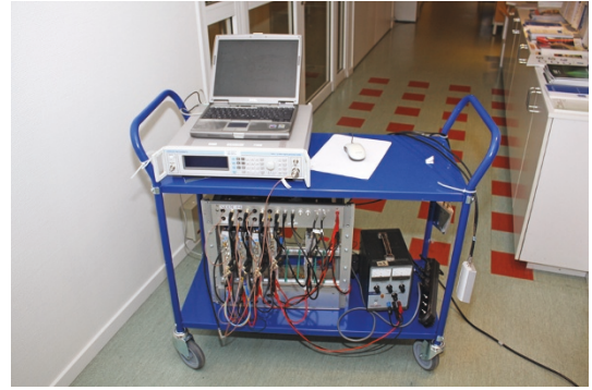
FIGURE 11: Node in corridor.
