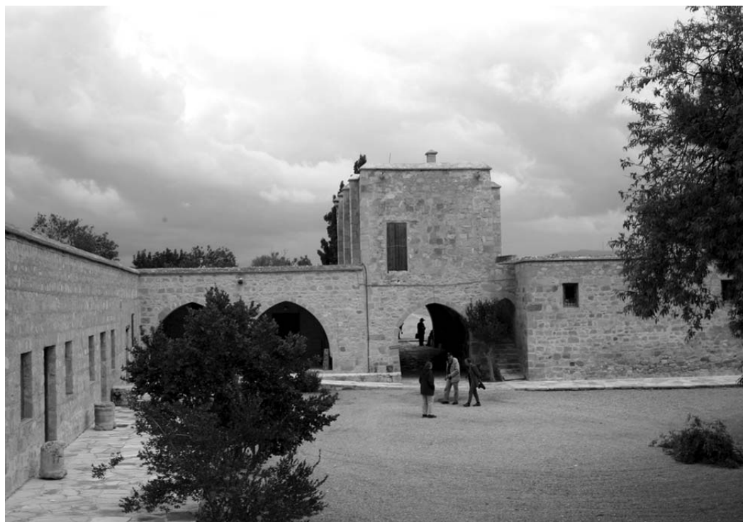
Figure 3 Courtyard of reconstructed manor house of Koukklia, with two-storey entrance tower
