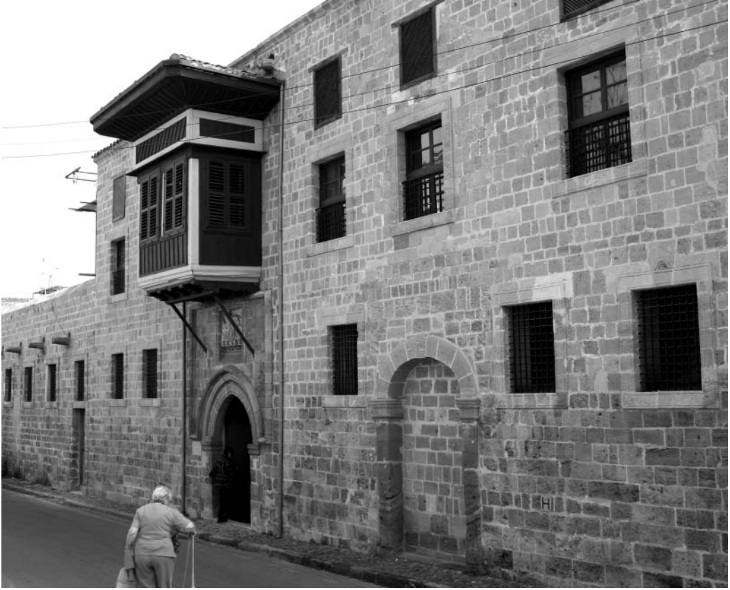
Figure 2 Façade of the konak of Hadjigeorgakis Kornosios, with entrance, marble plaque and projecting window
