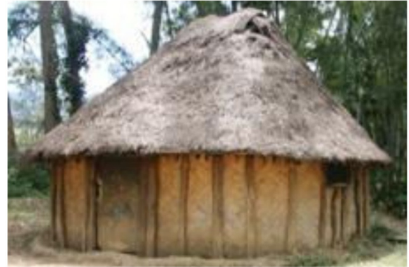
Figure 3 A traditional housing structure in Masumave, PNG Highlands.
