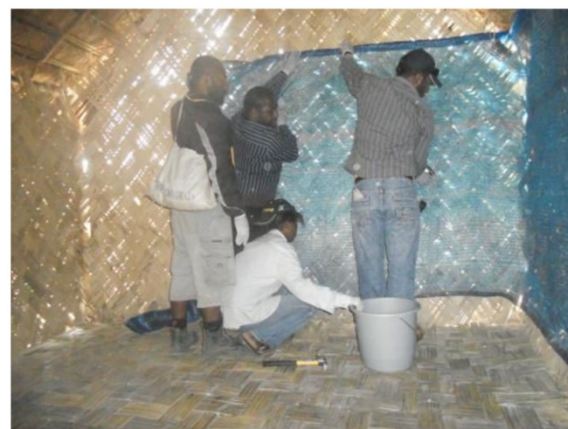
Figure 5 Installing ZeroVector® ITPS in a Highlands village house.
