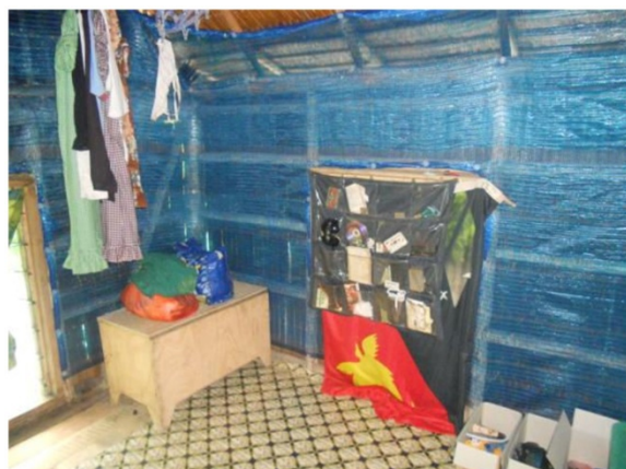
Figure 6 The interior wall of an Islands village house four-weeks post ZeroVector® ITPS installation.
