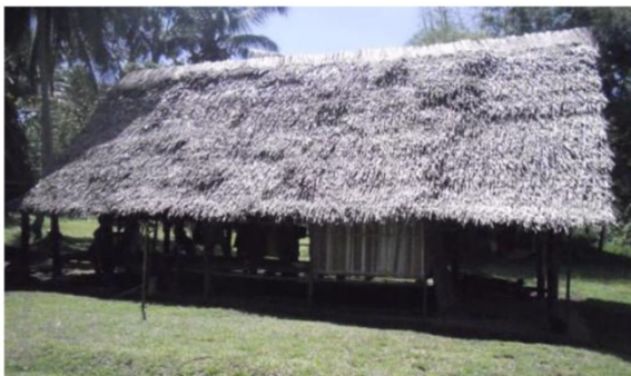
Figure 2 A traditional housing structure in Nauna, PNG lowlands.
