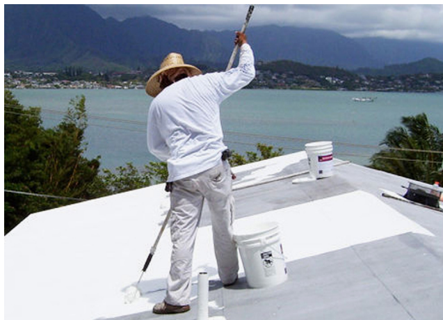
Figure 10 Reflective white roof paint (Cool Roof Hawaii, 2013).
