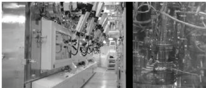
Fig.10.Appearance of TRU-HITEC and electrorefiner for Am and Cm bearing nitrides.
