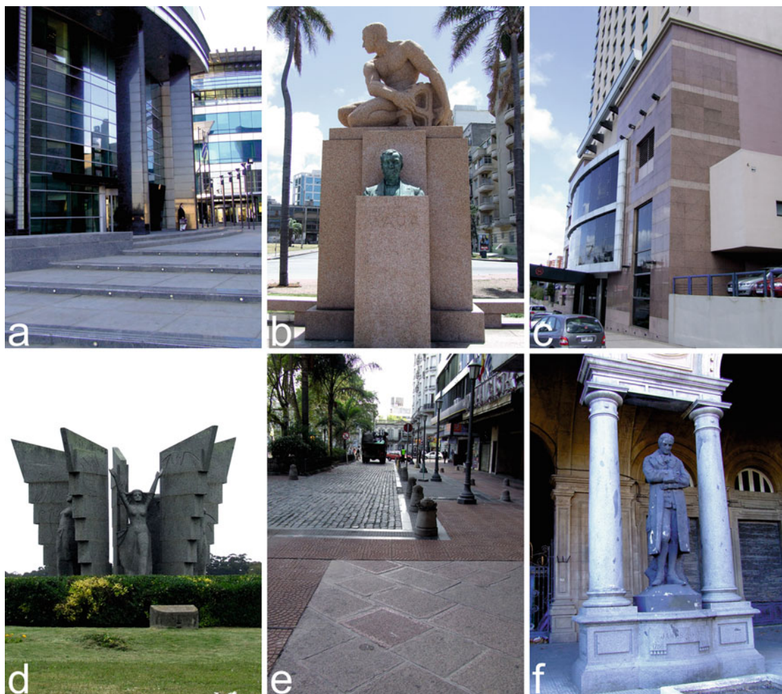
Fig. 1 Uses of Uruguayan commercial granites in the city of Montevideo; a outdoor façade cladding using Moderate Black Dolerite and flooring slabs using Cufre Granite in the Antel Tower; b outdoor sculpture (Vizconde de Mauá) using La Paz Granite; c outdoor façade cladding using polished and unpolished slabs of
