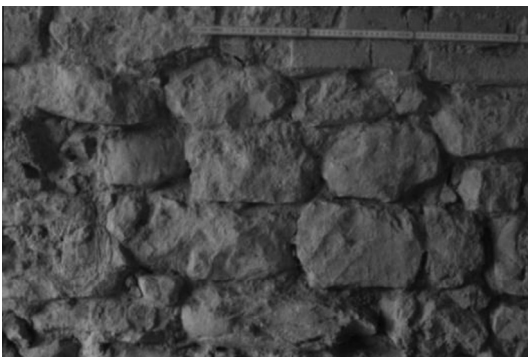
Fig. 7. Stonework of Colle Umberto farm house (20th-century).
