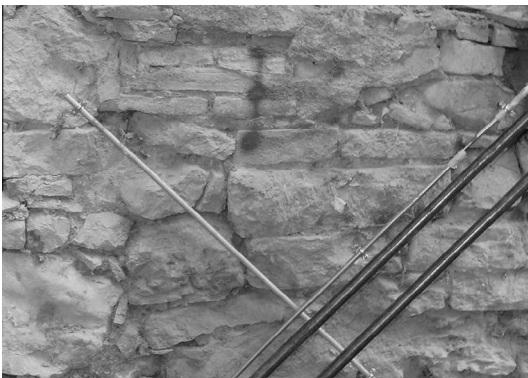
Fig. 6. Stonework of Colle Umberto farm house (19th-century).
