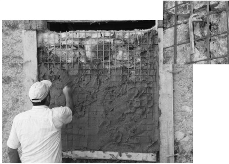
Fig. 5. Application of mortar jacketing and detail of connection between anchors and GFRP grid.
