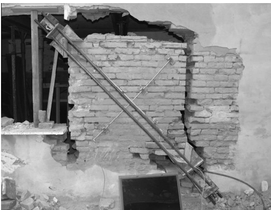
Fig. 1. On-site diagonal compression test (San Felice building).
