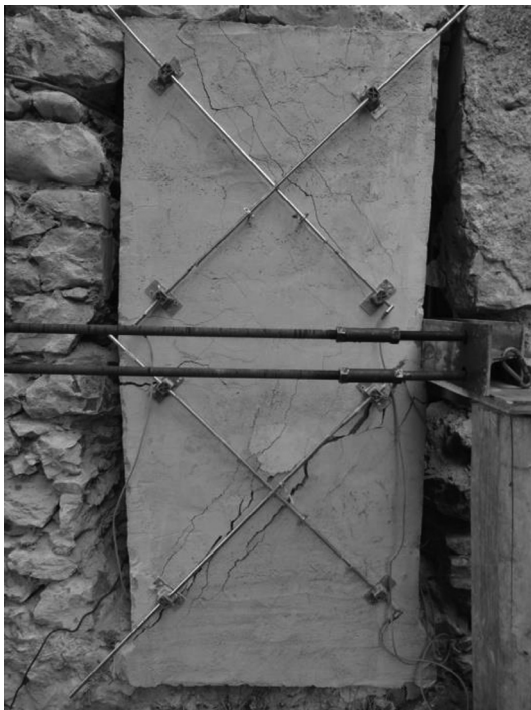
Fig. 14. Crack pattern of a reinforced wall panel tested at Colle Umberto.
