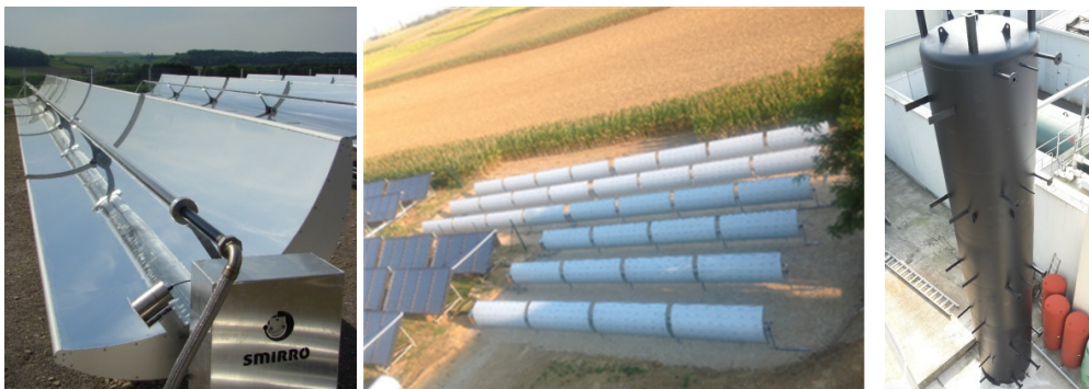
Fig. 2: Parabolic trough collector system installed at BERGER, Austria; (a) parabolic trough, (b) collector field, (c) 20 m 3 storage
