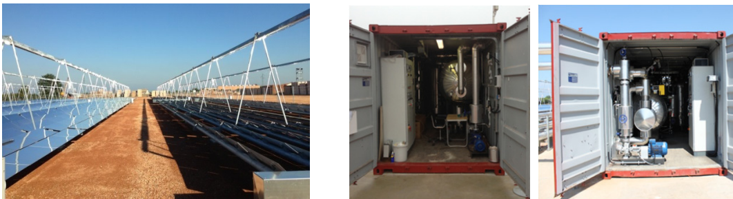
Fig. 4: Solar process heat system installed at Laterizi Gambettola SRL; (a) collector field, (b) and (c) B.O.P.'s
