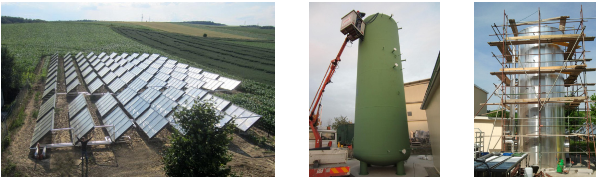
Fig. 1: Solar process heat system of SOLID installed at BERGER, Austria; (a) collector field; (b) storage installation; (d) final 60 m 3 storage
