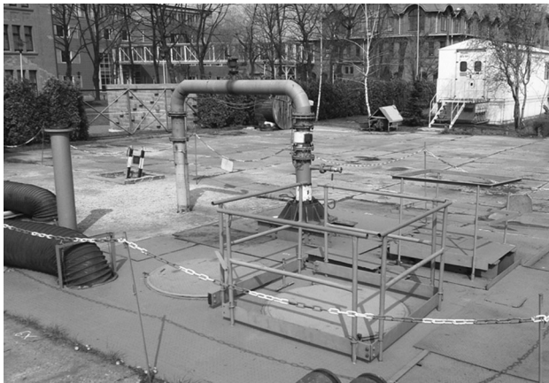
Fig. 1 Site—Gliwice II shaft which is located in a very urban environment
