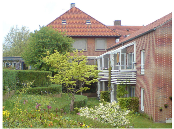
Fig. 9. Enclosure and entrance. Hedges and plantings in stages create enclosure without confining.
