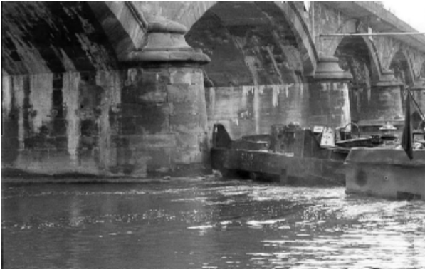
Figure 1 Ship impact against bridge.
