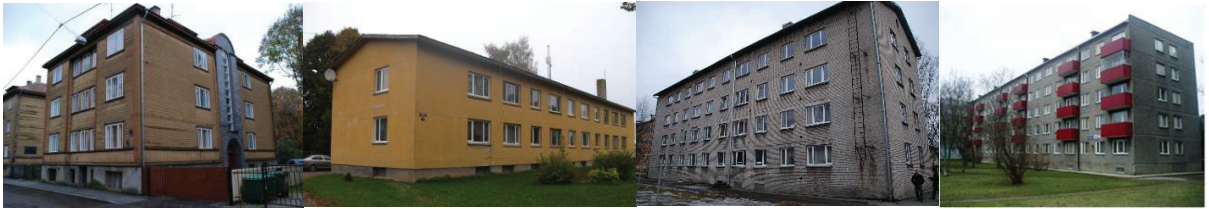
Fig 1. Main building types (from left to right): wood, large block, brick, and large panel.
