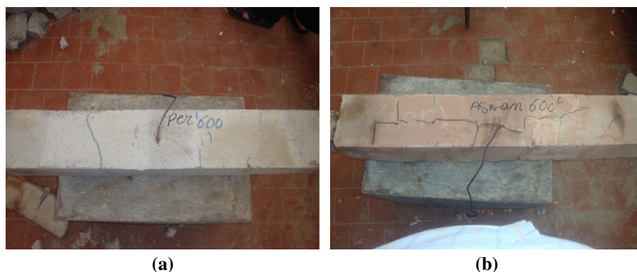
Fig. 10 FRP-strengthened RC beams protected by type 1 and 4 after exposure to 600 °C. (a) Beam protected by type 1 (Perlite mortar) (b) Beam protected by type 4 (Aswan clay).
