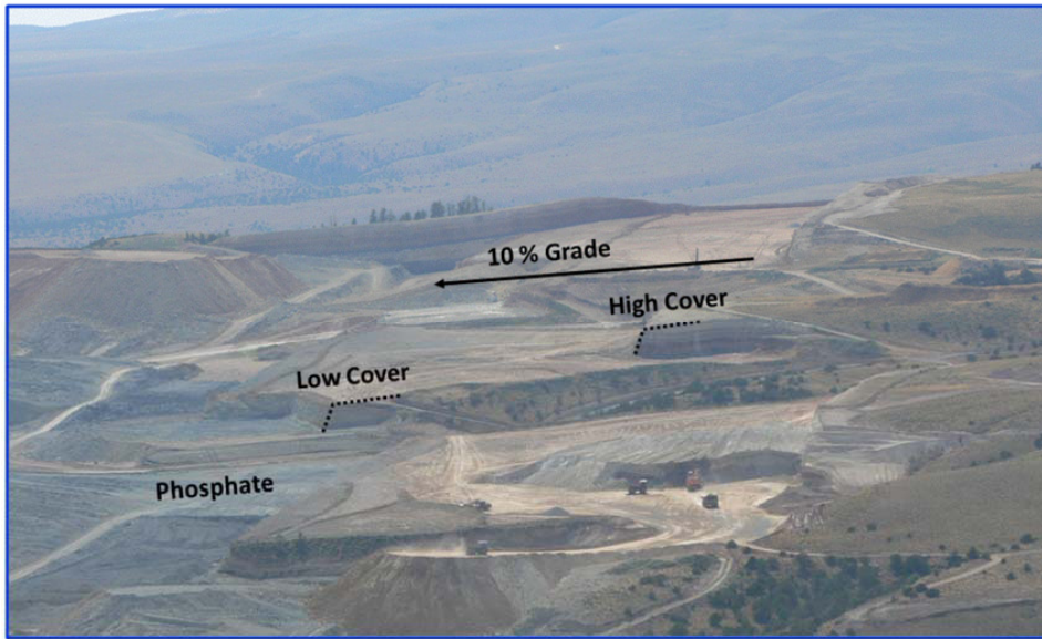
Fig.4: Three pass mining process, high cover, low cover and phosphate ore. (Mc Allister and al., 2012)
