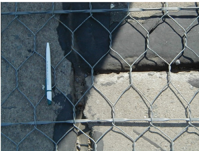
Fig. 2. Steel reinforcing mesh.
