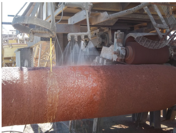
Figure 4 Concrete mix using local hematite aggregate during application by impingement machine.
