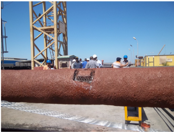
Figure 6 Coupon sample from the concrete coating local hematite around the pipe.
