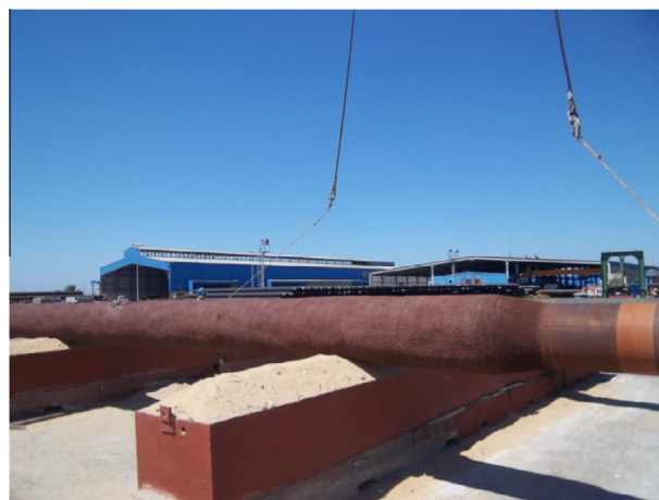
Figure 5 Concrete mix using local hematite aggregate after application on pipe.
