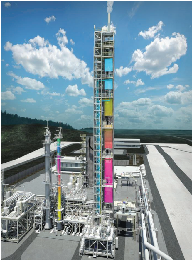
Figure 1 : Absorber and regeneration units in the amine plant
