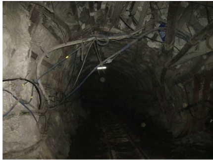
(a) The horizontal and vertical directions are in high stress level and the whole section shrinks.
