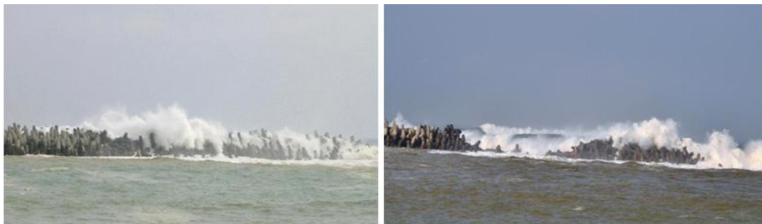
Fig. 3. The breakwater head is badly destroyed by strong waves (left: before the destruction; right: after the destruction)
