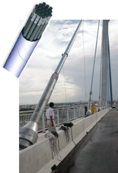
Figure 4. Measurement of cable vibration at Phú Mỹ Bridge
