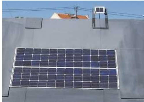
Fig. 3. PV system formed by two monocrystalline solar modules connected in series [8].
