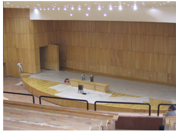
Figure 7 Absorbing low frequencies utilizing membrane absorber.
