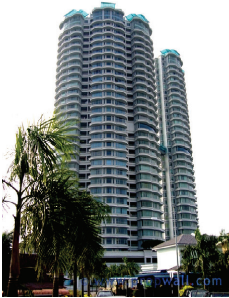
Fig. 4. The View residential building, Penang
