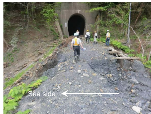
Fig. 7. Tsunami-induced damage to embankment along North Rias line of Sanriku Railway between Shimanokoshi and Tanohata stations (adjacent to Hiraiga tunnel).
