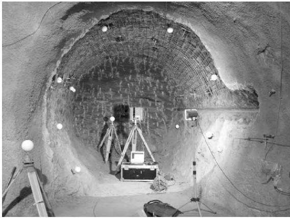
Fig. 3 Laser scanning of excavation surface of tunnel
