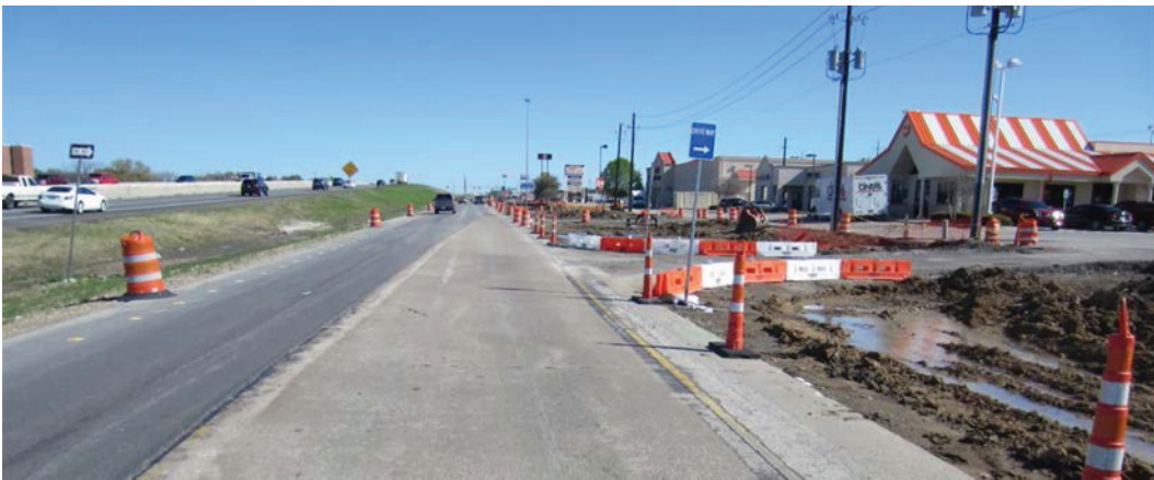
Fig. 2. Treatment 2: 42-inch cones with 18-inch LCD.
