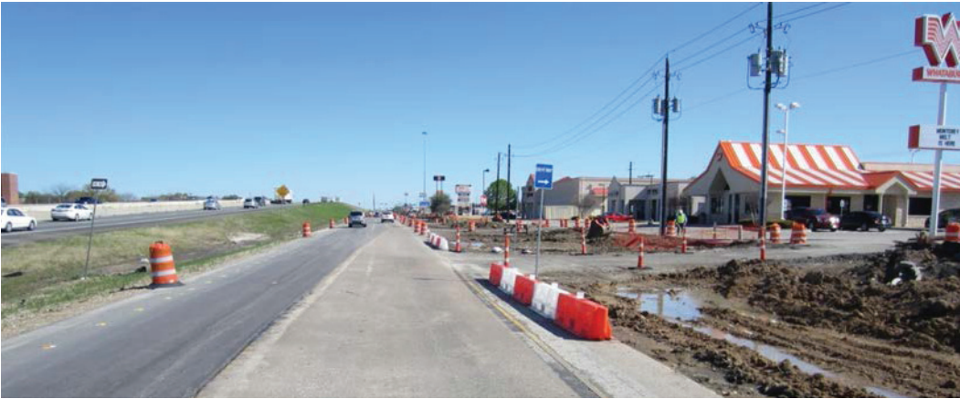
Fig. 1. Treatment 1: 18-inch LCD with 42-inch cones.
