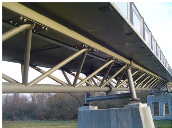
Fig. 1 Gärtnerplatzbridge in Kassel, Germany (2007), consisting of a high performance deck glued to a 3-D steel truss
