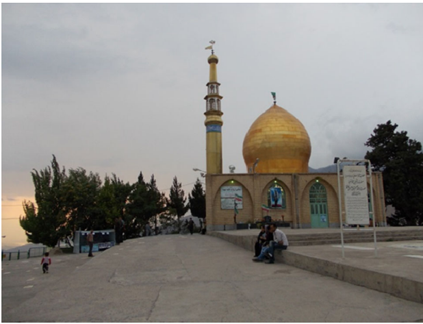
Fig. 1 Shrine of an Imam Zadeh—a pilgrimage place—near the Rudbar-Manjil area. Photograph by M. Ibrion, 2012
