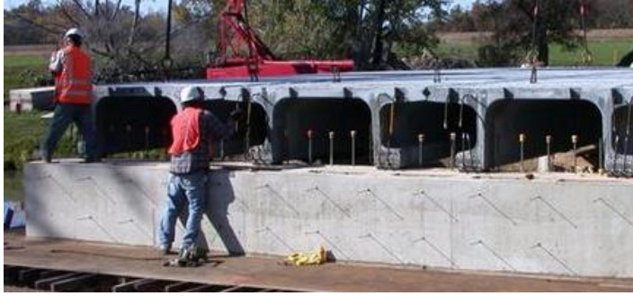
Figure 2: Optimised UHPC bridge girder design [19, 20].
