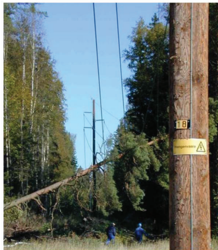
Fig. 4.6. A tree is falling on the CC lines passing through forests [95].
