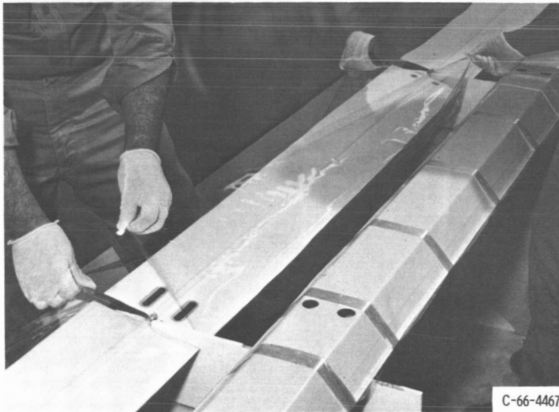
Figure 19. - Packaging operation showing protective plastic sheeting and stiffening members being placed on fins after spray coating.
