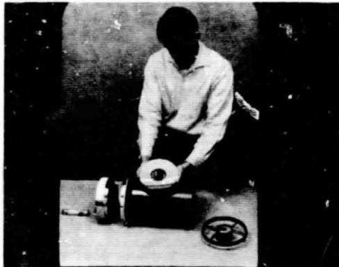
FIGURE 3. RANGER TELESCOPE DISASSEMBLED
