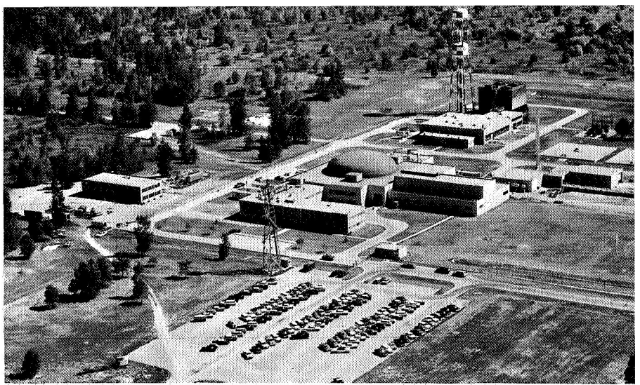
This shows the Plum Brook 60-megawatt research reactor facility. Built on a 6,000-acre site, the reactor is being used for numerous basic physics, materials and components tests leading to the development of a nuclear rocket engine system.
