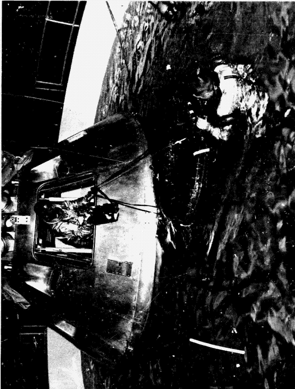
Figure 7. - Egress testing - Main crew hatch test tank facility.
