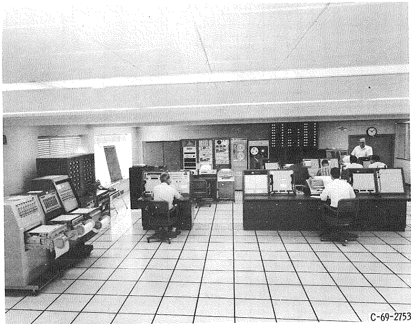
Figure 4. - SERT II control center.
