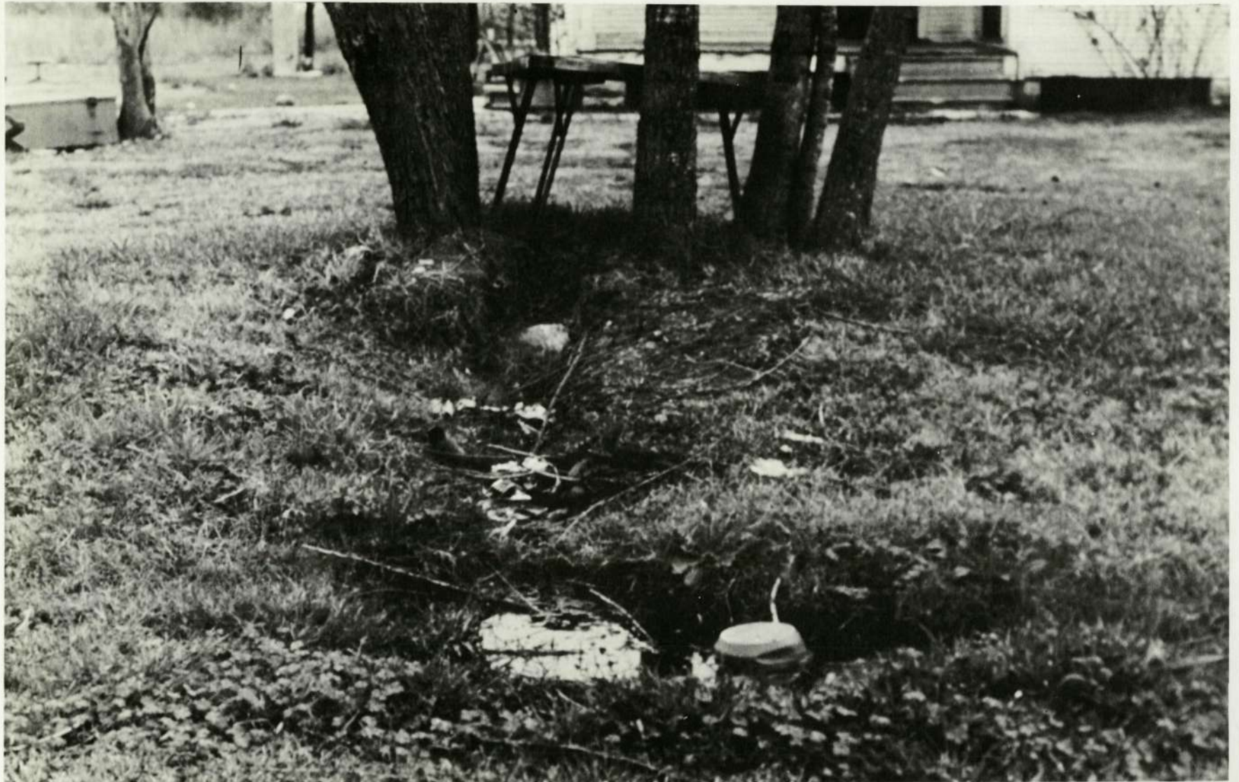
Figure 4.- The effluent from septic tanks in thousands of adjacent homes, unable to percolate thru the hard pan, flows thru pipes to openings near these collecting ditches. In this figure we see septic tank effluent running from a pipe opening in front of the trees in the front yard of this house.
