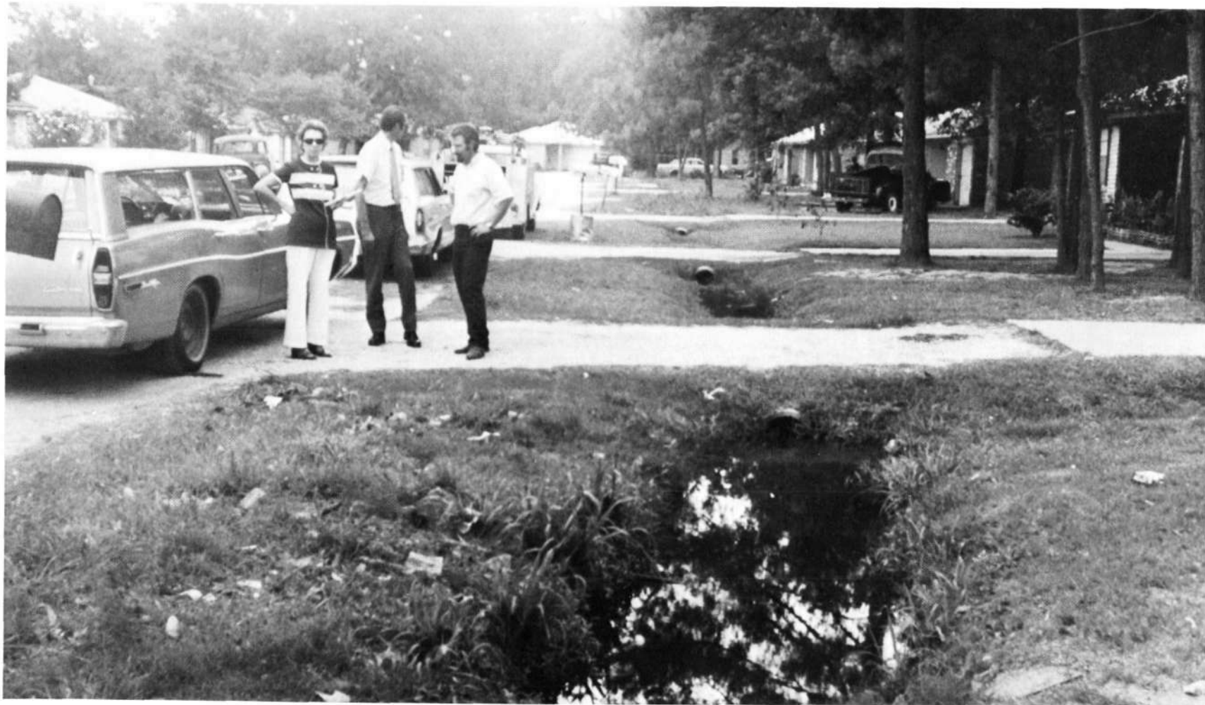
Figure 5.- This collecting ditch is representative of some 1,600 miles of collecting ditches in Harris County. Approximately $900,000 are required each year to find and control Culex quinquefasciatus larvae in Harris County, Houston, Texas.
