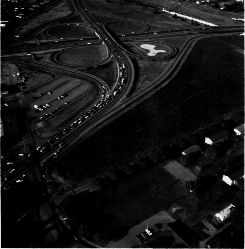
FIGURE 50.—A sample photograph showing how low-level aerial photography might be used for traffic engineering analysis in evaluating flow patterns, delays and behavior of drivers at converging lanes. If one looks closely enough at the photograph, where the feeder lane converges from the viewer's left into the stream of traffic moving downward into the left, one can see a car tailgated bumper-to-bumper to prevent traffic from merging.
