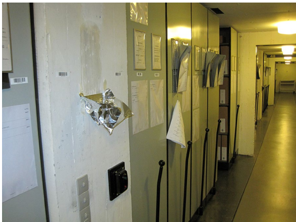
Fig. 3 The Koppel Wing of the Danish State Archives from the 1960's, where concrete was the dominant building material. On the left in the photo can be seen the sampling site with the Al-foil still in place (photo: Morten Ryhl-Svendsen)
