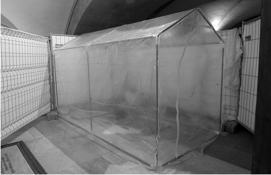
Fig. 2. The special on-site climate-control chamber built over the entrance of the crypt to maintain the humidity and temperature inside.
