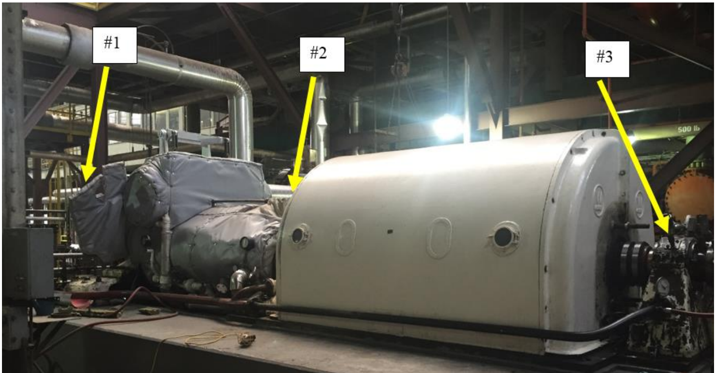
Figure 10 - Turbine Generator Balance/Measurement Planes
